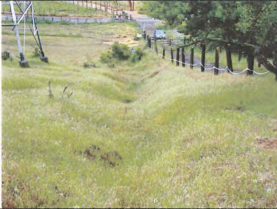
Photo 1. View to the south of the incised drainage ditch along the western fence line.
