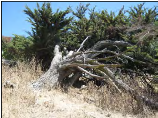
Photo 1: 35" Monterey cypress has failed and should be removed.
