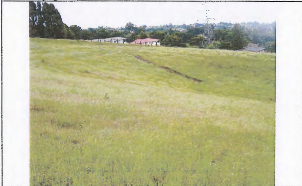
Photo 6. View to the south of the hillside containing the potential seasonal wetland seep.
