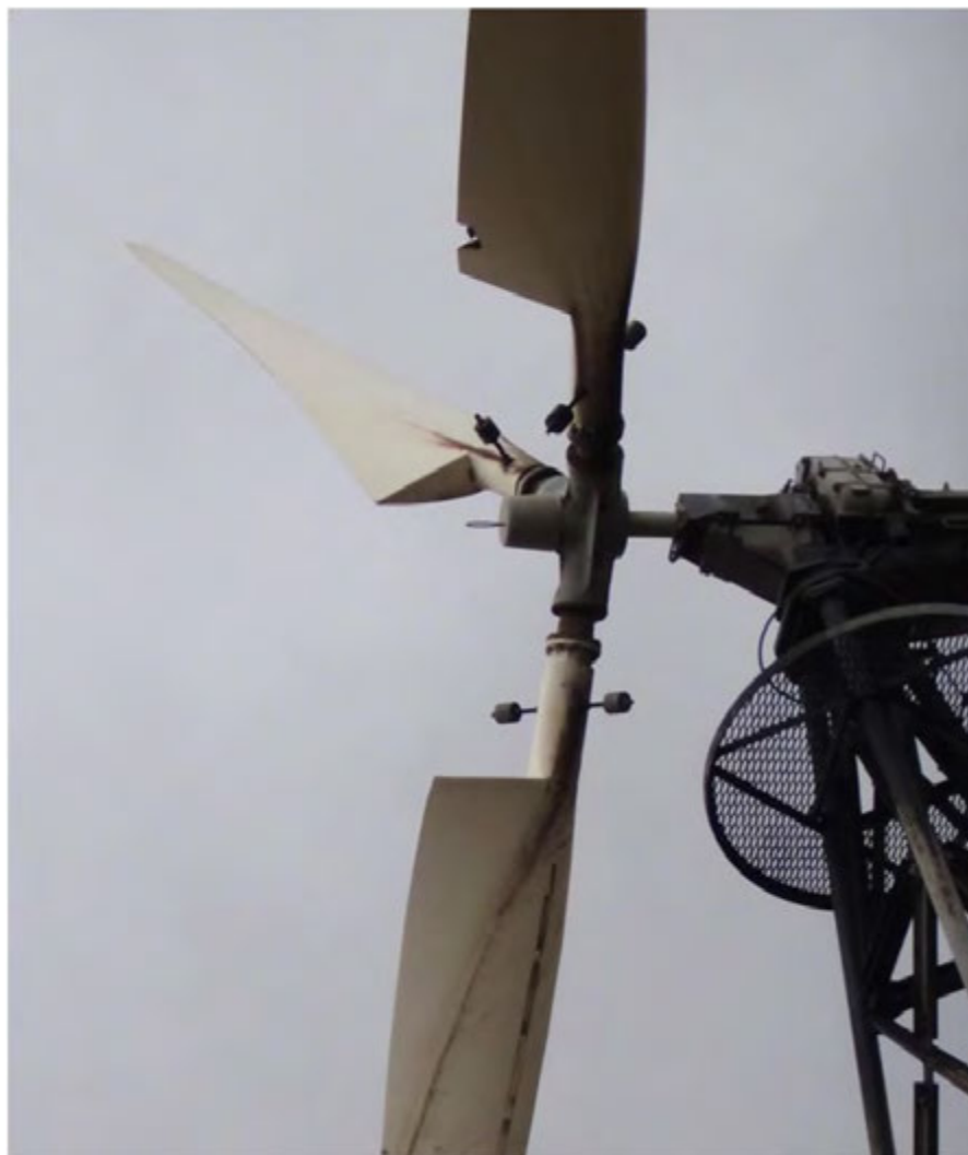
FIGURE 4 CLOSE-UP VIEW OF RUST STAINING EMANATING FROM WIND TURBINE IFD ROD
